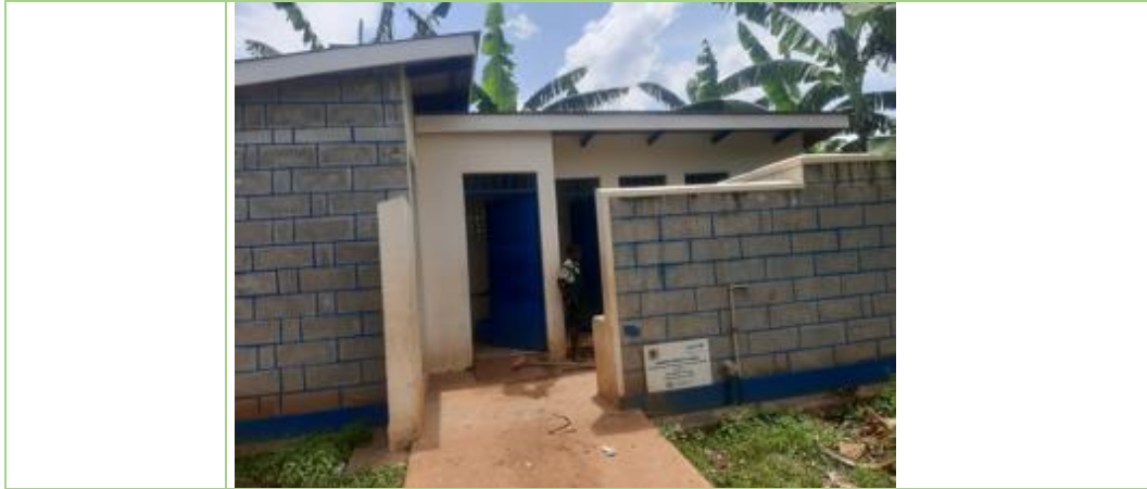
Figure 57: A Separate Five Stances Drainable Latrine for Girls with a Changing Room with Water, a Disposal Bucket, Sanitary Towels and Soap
