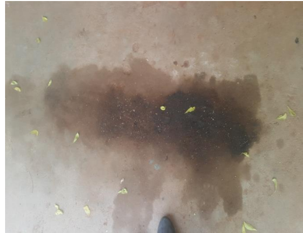
Figure 49: Oil spills outside the mechanics workshop
