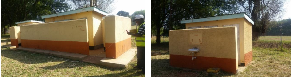
Figure 18: Pit latrines and bathroom
