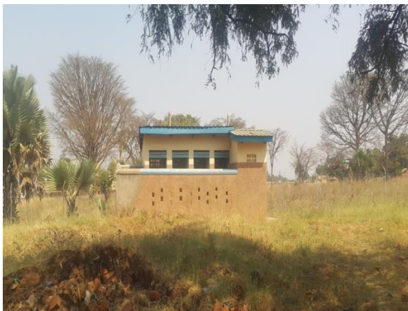
Figure 44: New sanitary facilities
