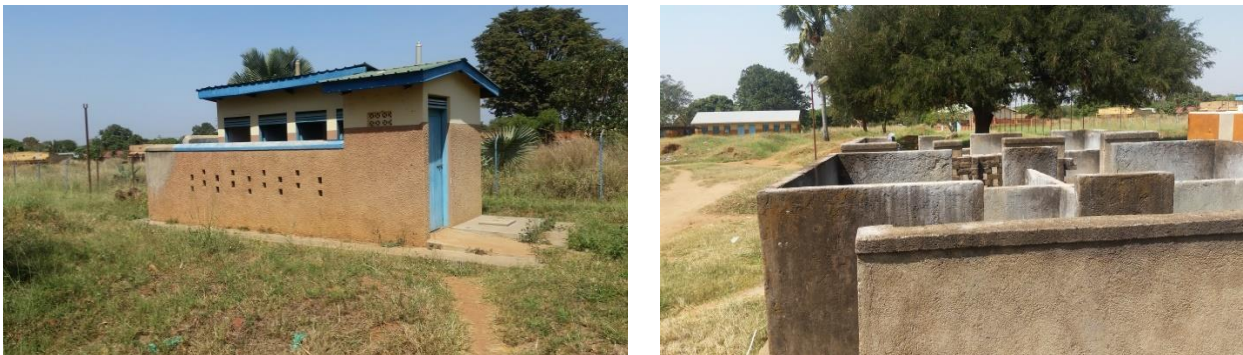
Figure 19: Standalone pit latrine & Bathrooms
