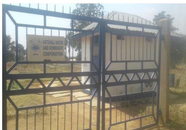
Figure 41: NWSC service station under construction at the institute
