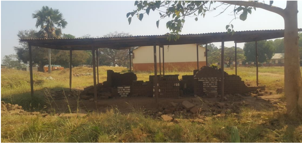
Figure 36: Building construction workshop
