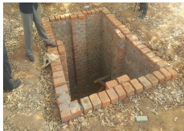
Figure 47: Septic tank under construction by Building Construction students
