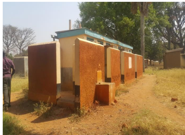
Figure 45: Facilities at the boys' dormitories
