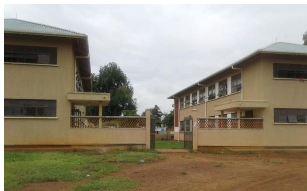
Figure 18: New Boys' dormitory building
