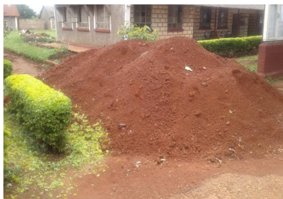
Figure 28: Construction material stockpiles
