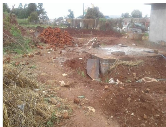
Figure 24: Foundation laying for another structure
