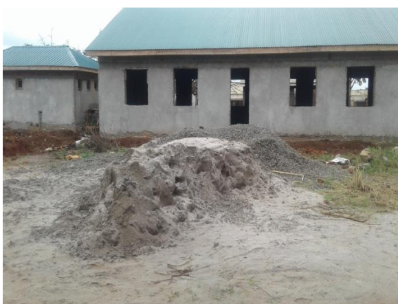
Figure 23: Nearly completed Commercial structures
