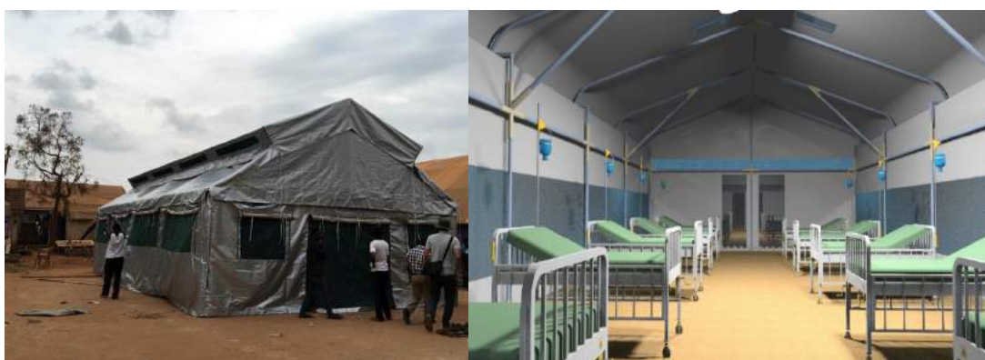
Figure 5.6.2.1. (c) EPI-TENT EXTERIOR
