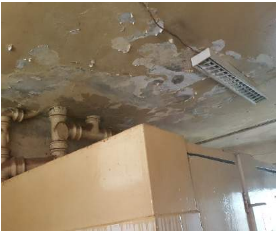
Leaking floor in Mitchell Hall
